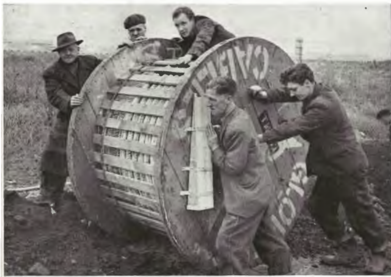
Pushing out the cable. Messrs. S. Barrow, M. J. Dunne, T. J. Stanton, H. C. McCarthy, and J. Milhench, working as a team somewhere in the wilds of the District. Phew! Warm work!
